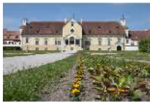
SAS.I, Ostfassade, DI014465, BSV
