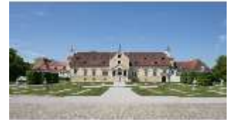
SAS.I, Ostfassade, DI014464, BSV
