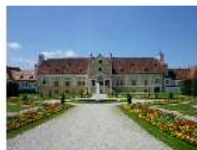
SAS.I, West-Fassade, DI009737, BSV
